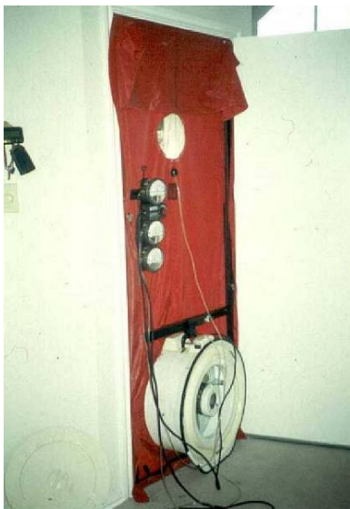
Figure 1. Blower door testing for building envelope leaks
