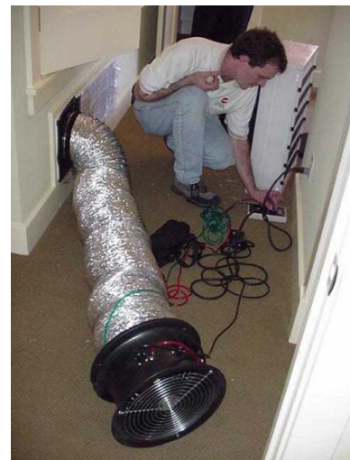
Figure 2. Testing for duct leakage
